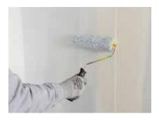
Gyproc Drywall Primer is applied to the entire board surface and jointed areas, to prepare the lining for final decorative treatment.
